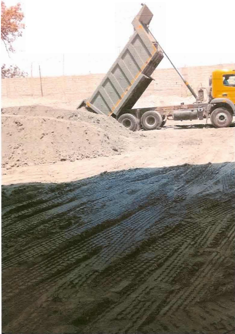
Unloading of Fly Ash
