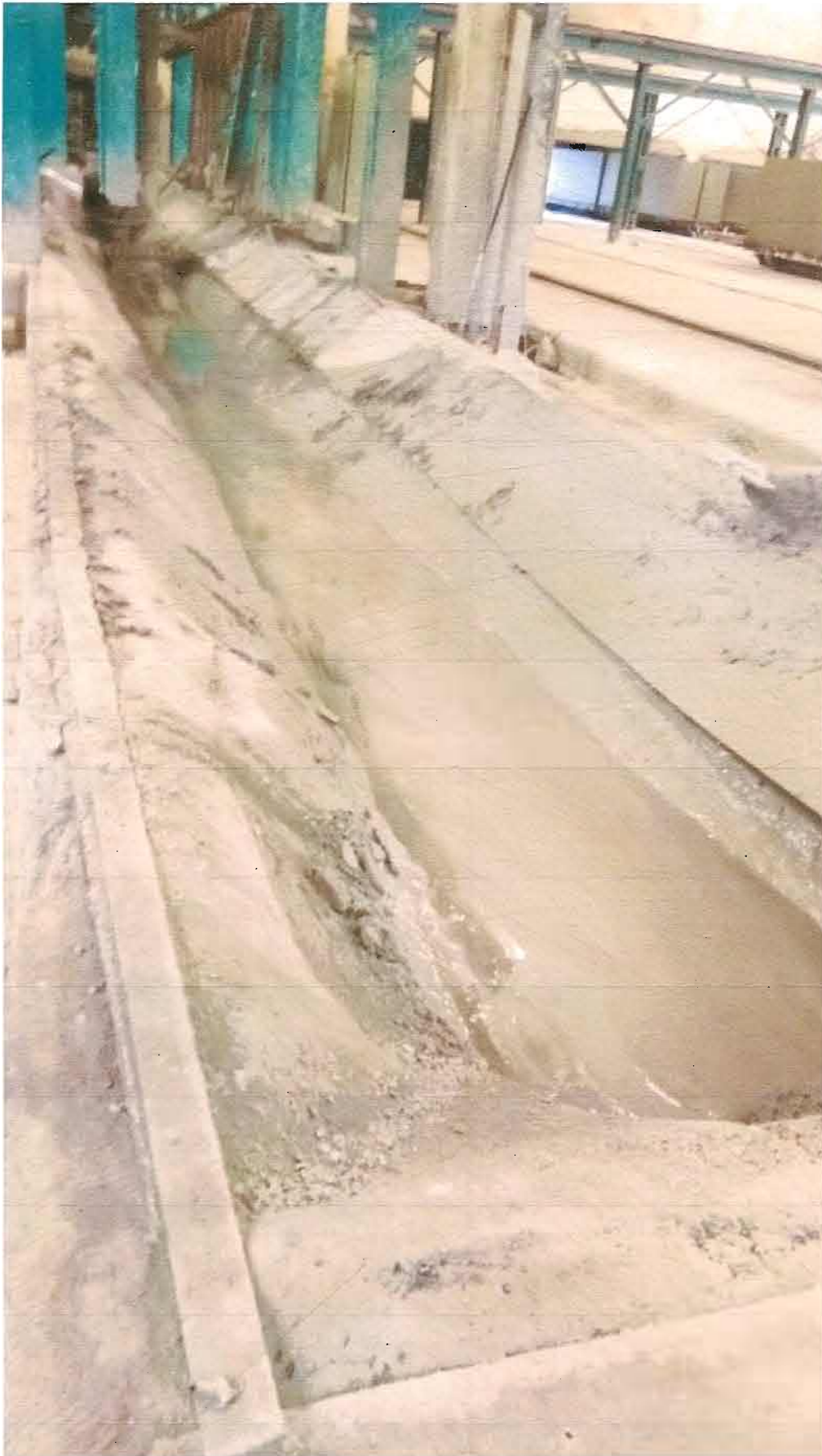
Leachate of fly ash
