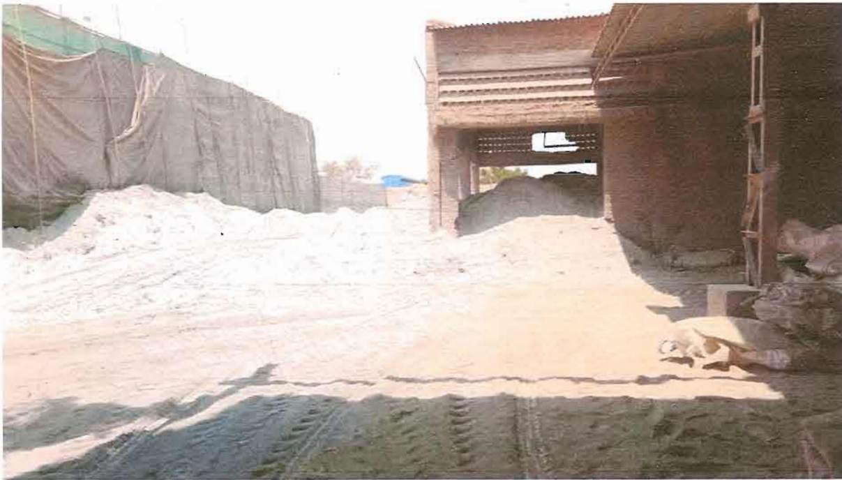
Fly Ash spread in the unit premises and source of mixing in the air
